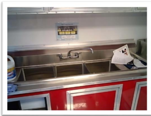
Three-compartment sink
